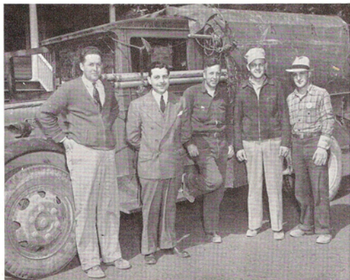
Part of the C. & K. force get final instructions before starting day's work at Rheem's shipyard. Left to right, Arthur Andrews, General Foreman; Mr. Kelman, Earl Mont, Assistant Foreman; George Skirrow and John McCann.
